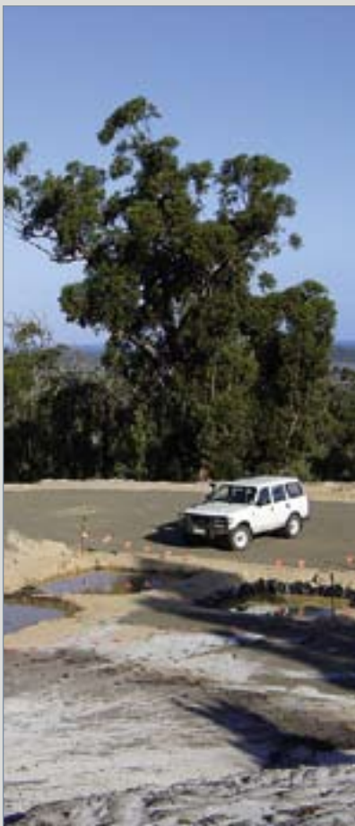
Site preparation at Banjo
